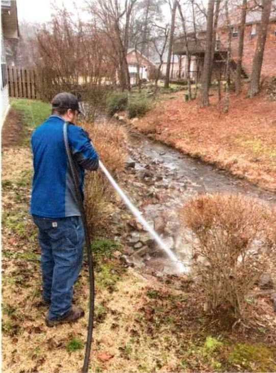
Manhole 3728 – 107 Forest View Court During Cleanup
