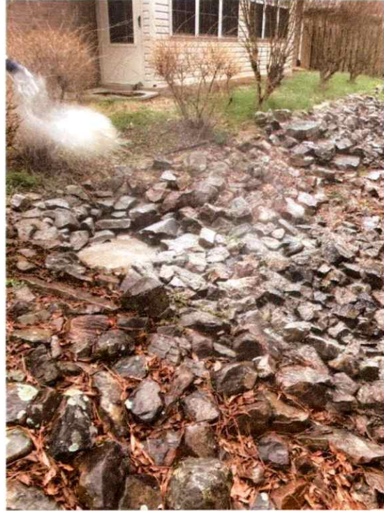
Manhole 3728 – 107 Forest View Court During Cleanup
