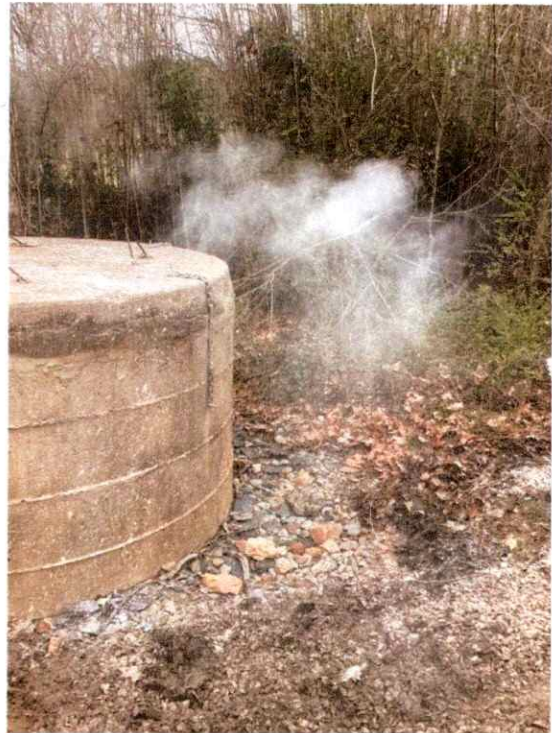
Manhole 1865 - 352 Fontana Road During Cleanup
