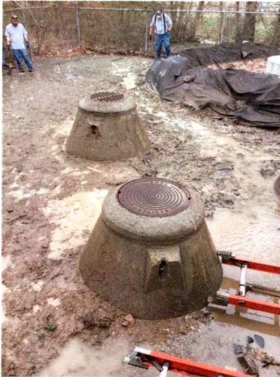
Manhole 1866 / HS Creek Pump Station - 362 Fontana Road Before Cleanup
