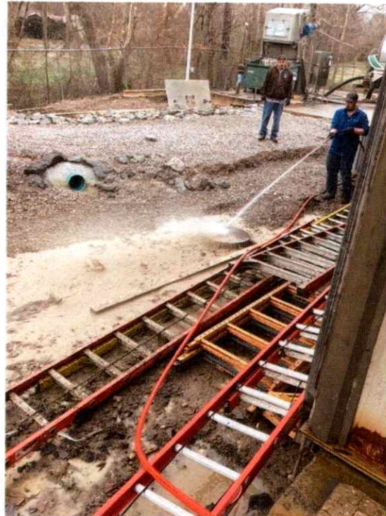
Manhole 1866 / HS Creek Pump Station - 362 Fontana Road During Cleanup
