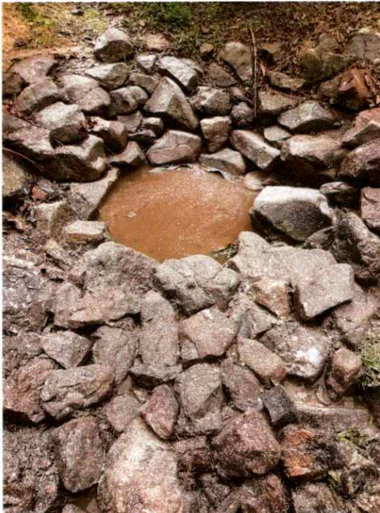
Manhole 3728 – 107 Forest View Court After Cleanup
