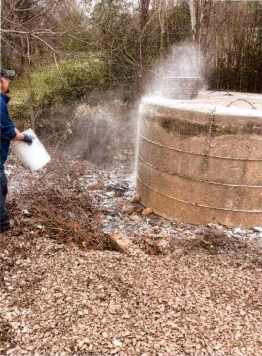
Manhole 1865 - 352 Fontana Road During Cleanup
